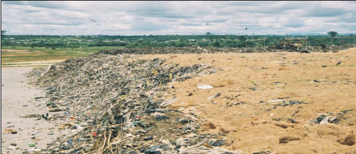
Plate 5-11: Daily Laterite soil coverage applied to waste at the Kumasi Landfill site
