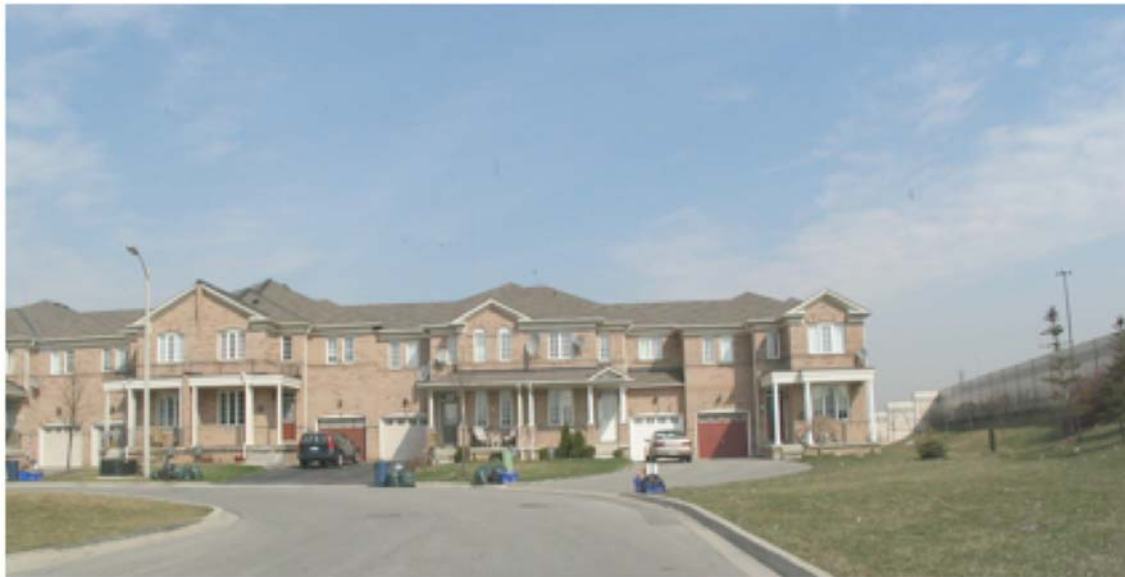
Figure 9.2: Peripheral row housing, Vaughan
