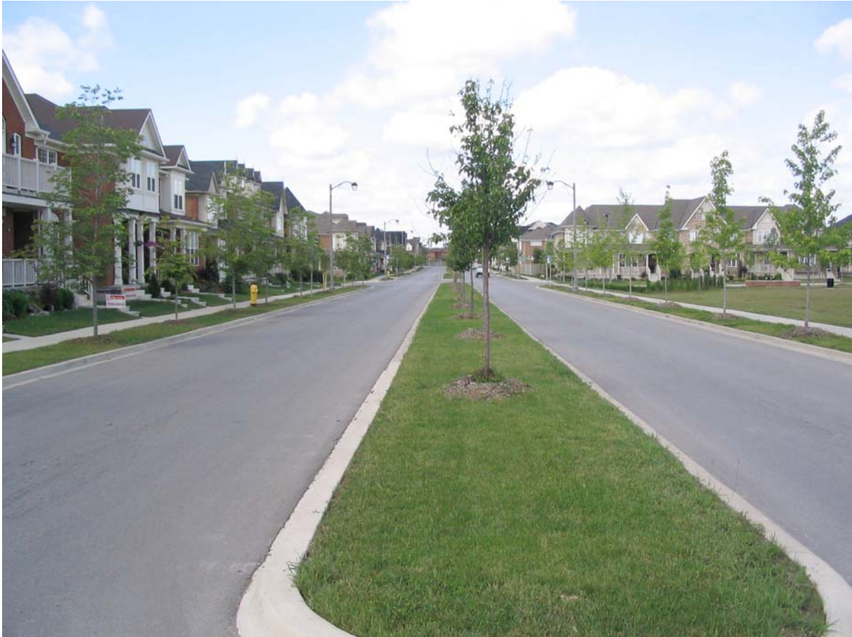
Figure 4.6: Oversized road in Cornell diminishes quality of pedestrian environment
