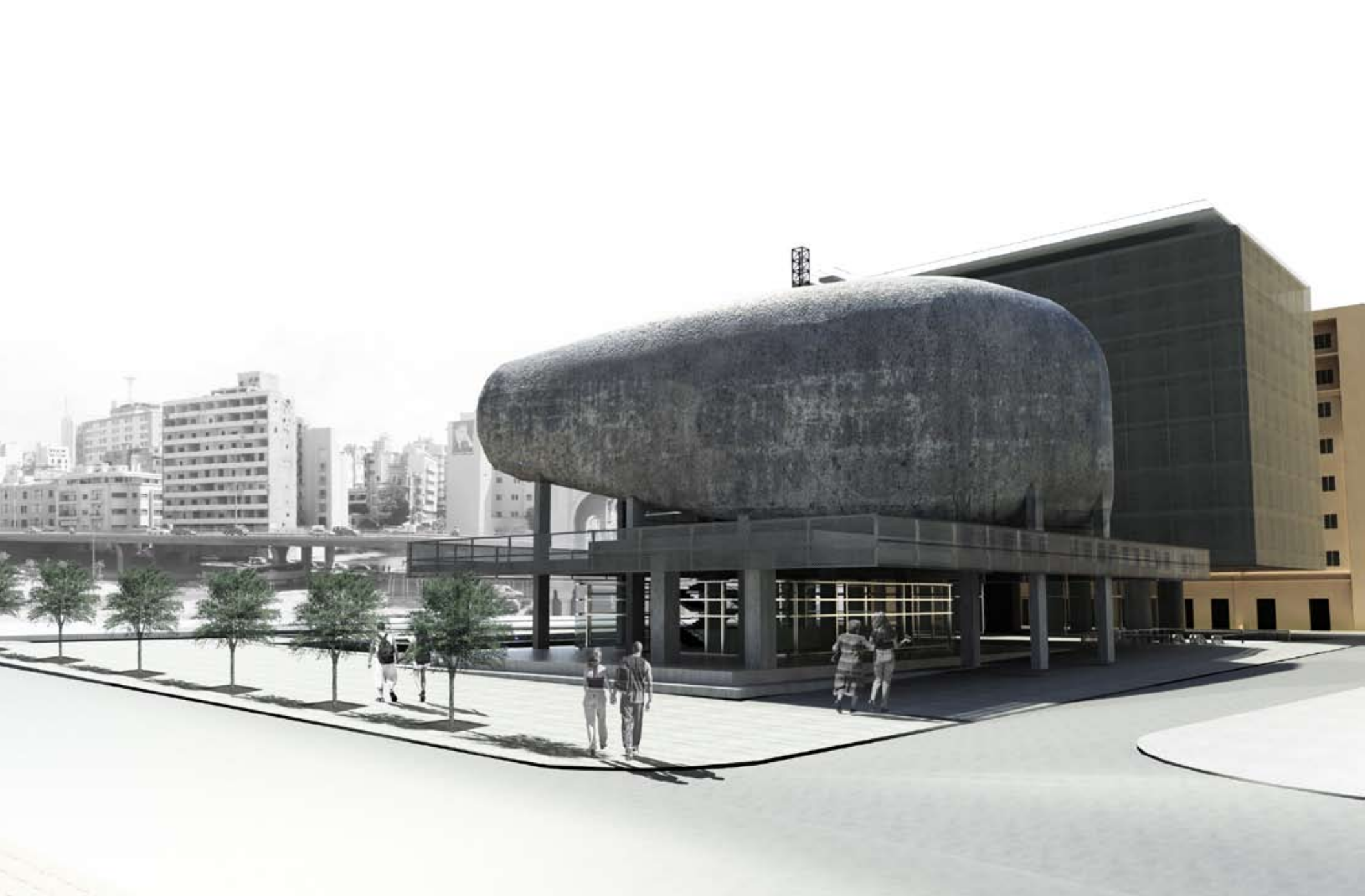
CCB . APPROACH FROM THE NORTH
