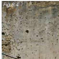
Rough cast concrete
