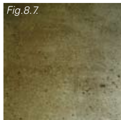
Fine cast floor concrete
