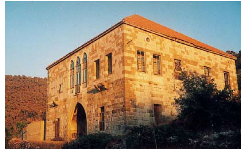
Fig.4.25. Image of a typical Central Hall House Type with a pitched terra-cotta roof. Photograph by Danny Noufaily.
