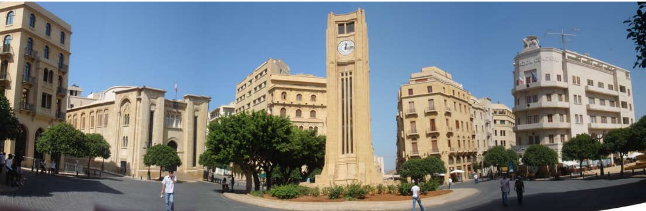
Fig. 6.4 Panoramic of Place de l'Etoile. The Lebanese parliament building is second from the left.
