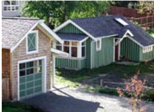
2.14 Cottage Housing Development “Backyard Neighbours” in Langley, Washington allows for an ADU apartment on the same lot as each small house in this new development.
