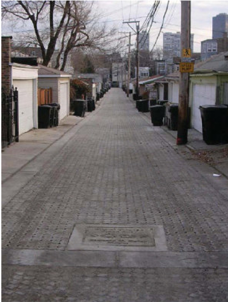
2.01 Recently updated laneway in Chicago, Illinois with an intricate paving pattern that also reduces stormwater runoff.
