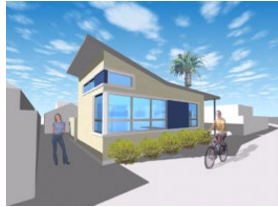
2.37 ADU prototype utilizes SIPs construction, a trombe wall and greywater storage and re-use. Design by CSS Architecture.
