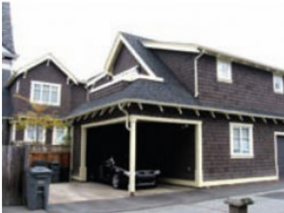
2.48 New laneway infill in Vancouver's Kingsway-Knight neighbourhood.
