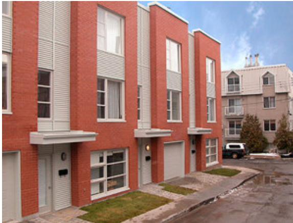
2.34 Les Lofts du Pont I , a five-unit infill project fronting on a laneway in downtown Montreal.
