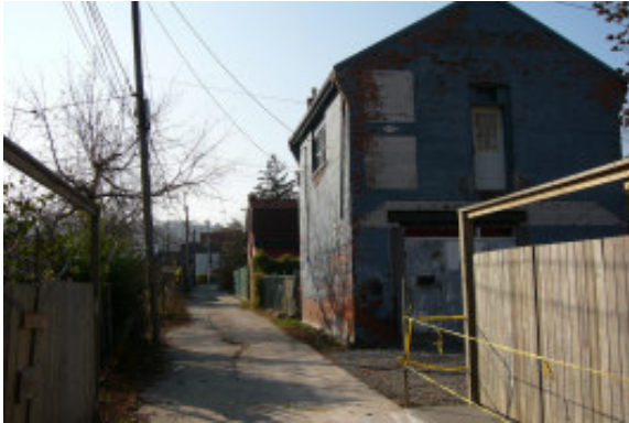
5.37 Existing converted coach house behind East Avenue North
