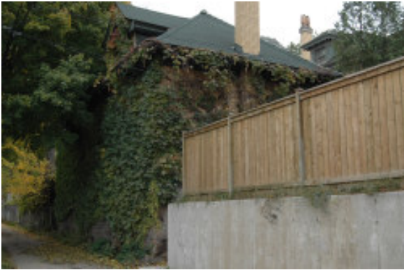
276 Aberdeen Avenue (rear apartments 1 & 2)
