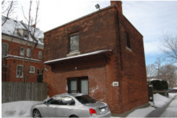
56 Charlton Ave. West (rear)
