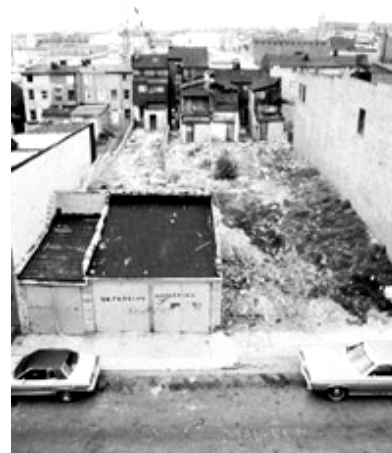
2.26 Chandlers Yard during construction in 1976. The three garages in the foreground were demolished and three rowhouses were infilled on the site.
