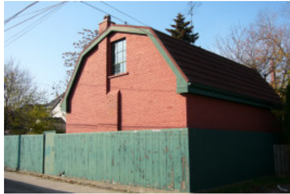
56 East Avenue North (rear)
