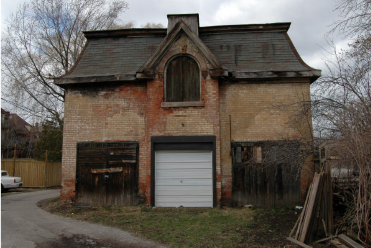
6.08 This vacant coach house in Hamilton's east end at 24 Blake Street holds great promise for conversion into a residence.
