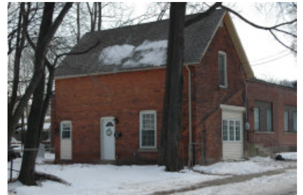
876 Main St. East (rear)
