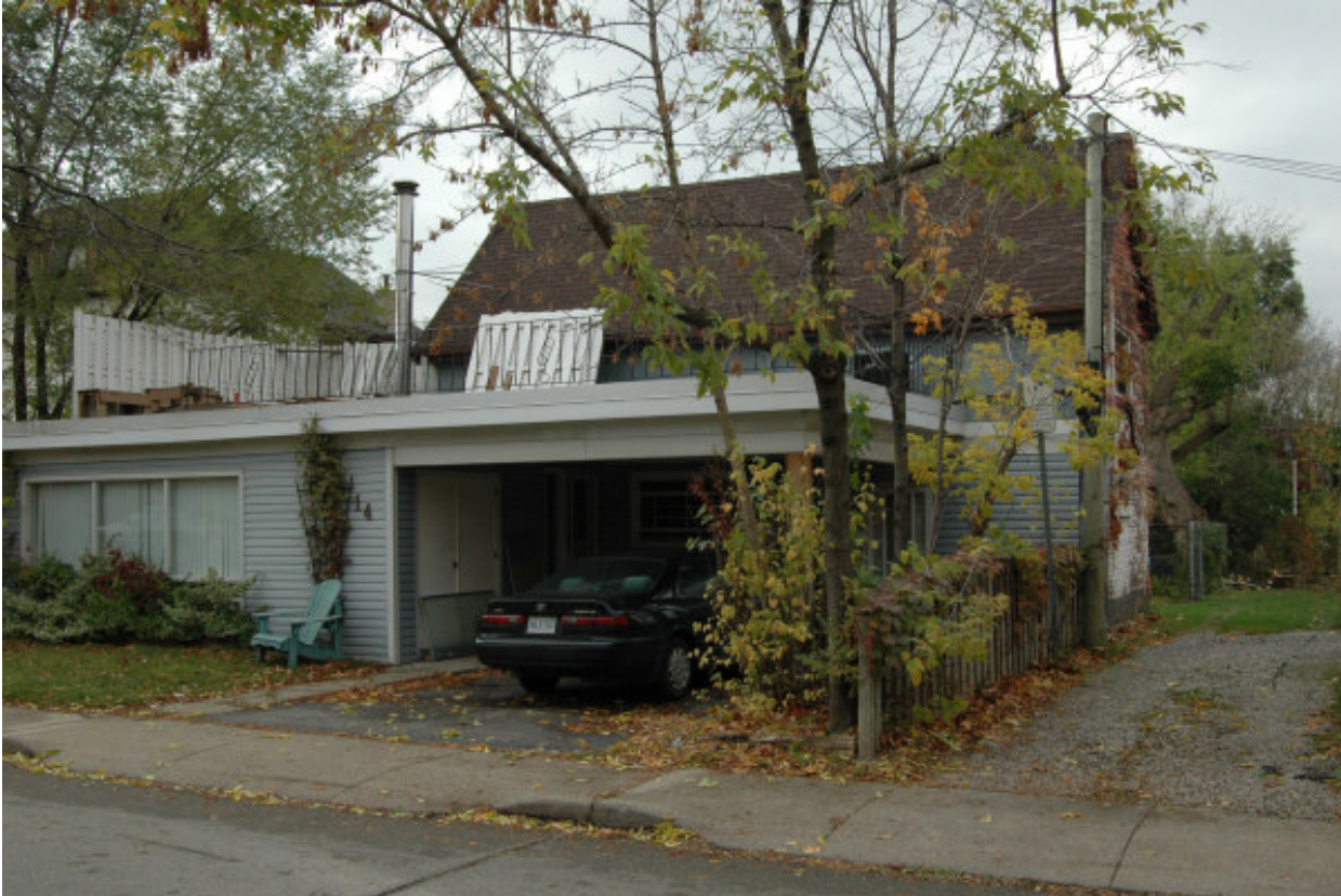
6.07 Converted coach house with a large addition at 14 Reginald Street, Hamilton.
