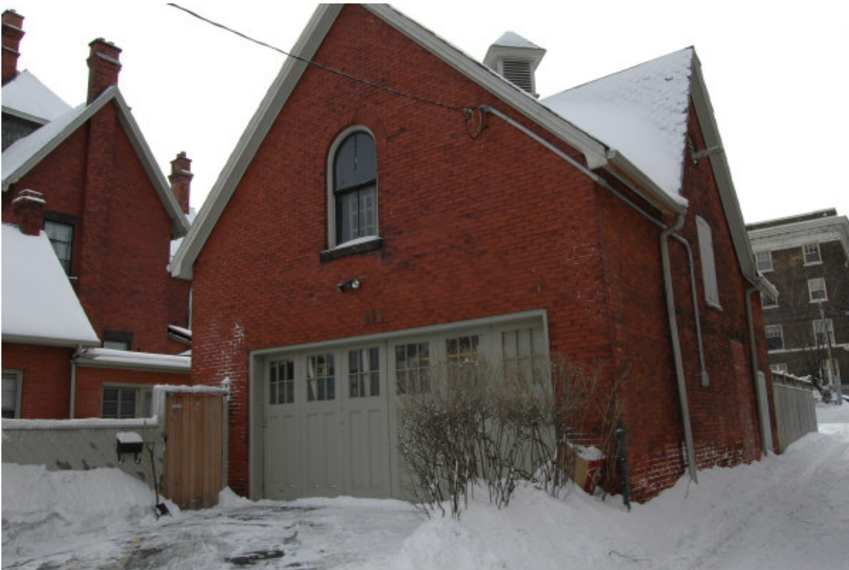
6.06 Large converted coach house in the Durand neighbourhood.
