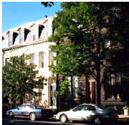
2.25 View of rowhouses on East Cross Street beside Chandlers Yard.
