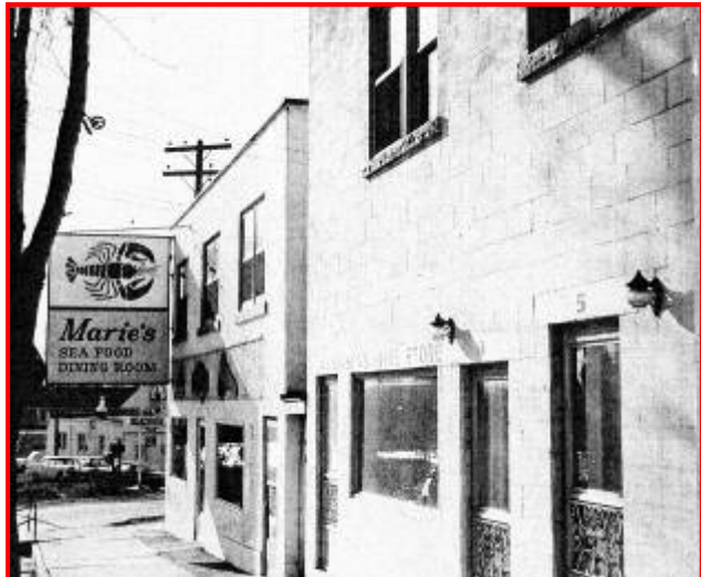
Lock Street, north of Front Street, 1969 Source: Salter (1969)
