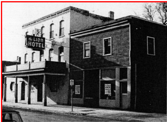
Wellington House later renamed the Lion Hotel dates back to 1877. Source: Aloian (1978)
