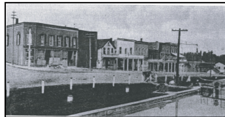
Figure 5.4: Old Front Street, 1905
