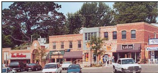
Figure 5.3: Old Front Street “echoed” in 50 Lakeport Road
