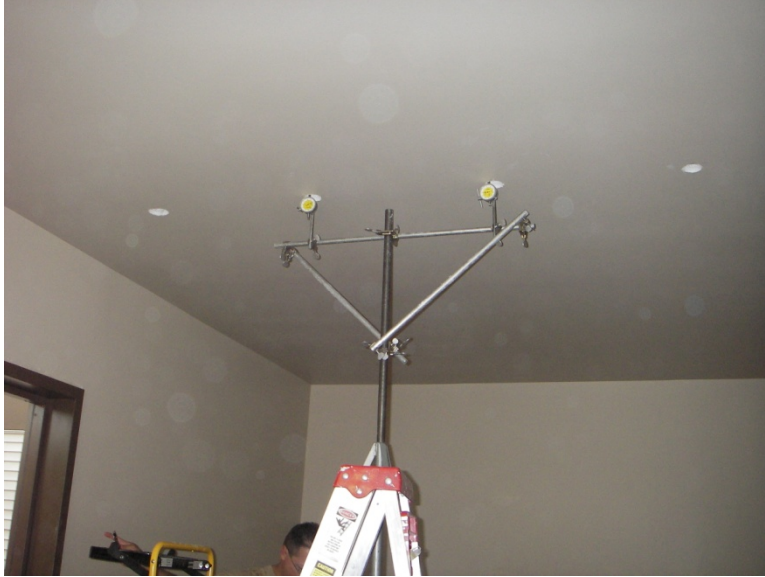
Figure 3-8: Drywall Openings for Joist Deflection Measurement
