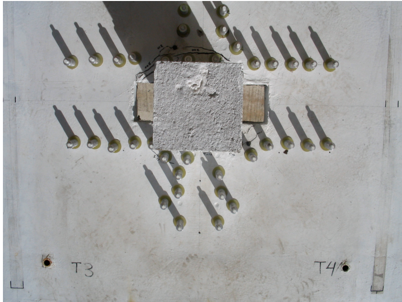
Figure 5.13 - Crack Pattern, Compression Side of Slab, SN6
