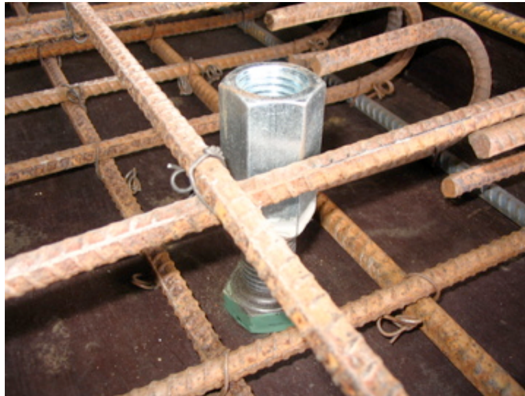
Figure 3.10 - Lifting anchor bolt prior to casting
