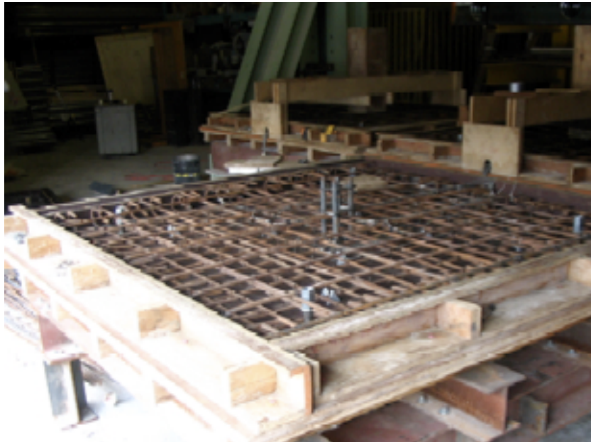
Figure 3.9 - Reinforcement Cages Prior to Casting
