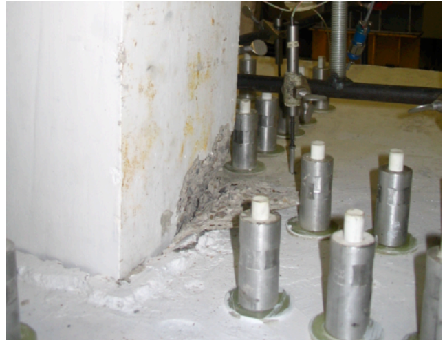
Figure 6.21 – Column Failure, SN5
