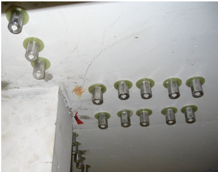
Figure 4.2 - K-Line Shear Bolts Installed in Slab During Testing
