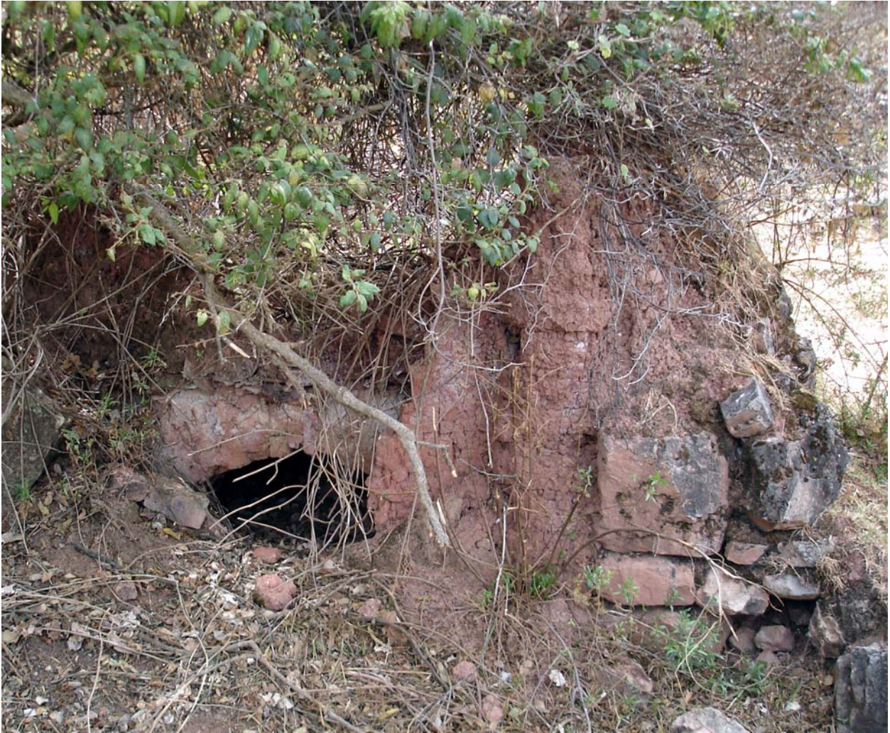
Figure 2. 29: Dwelling/structure of Acobamba village found buried within the rock/debris avalanche debris along the eastern boundary
