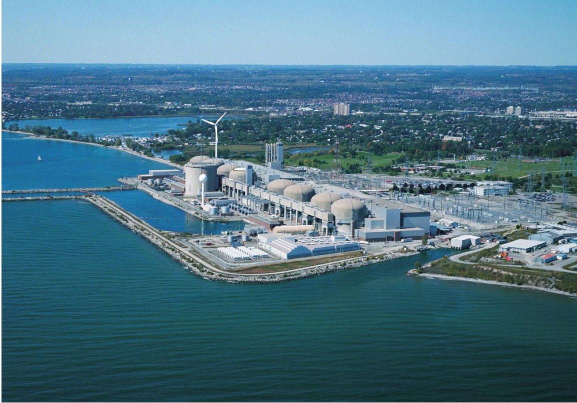
Figure 4-2 Aerial Photograph of the Pickering Nuclear Power Station
