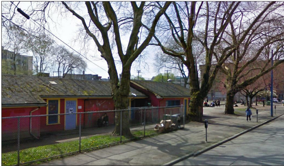
Existing Clubhouse is closed in-between scheduled activities
