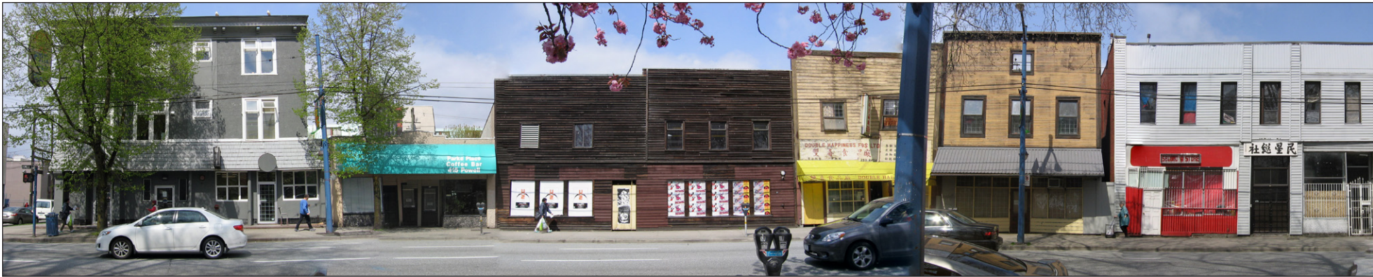
Fig. 3.17 Japantown Facades: Powell Street Elevation, across from Oppenheimer Park
