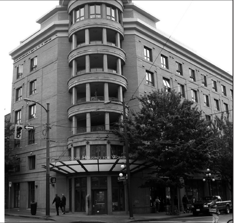
Bridge Housing for Women (home of DTES Women's Center and includes emergency housing for women)
