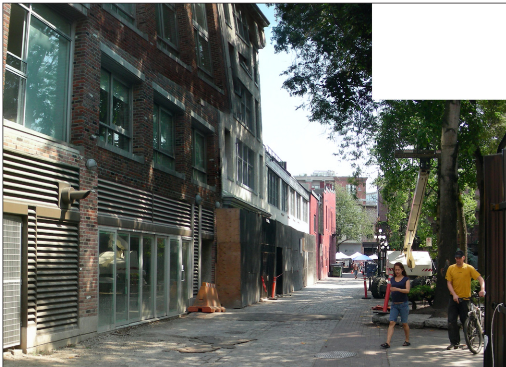
Fig. 3.34 Construction nears Completion, glazed storefronts face onto square
