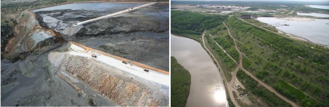
Figure 2.26. Spain's Tailing Ponds Break and a Tailing Pond near the Athabasca River (Source: Holroyd et al. (2009), "The Water That Bind Us: Transboundary Implications of Oil Sands Development," Pembina Institute, February 2009, p. 21.)
