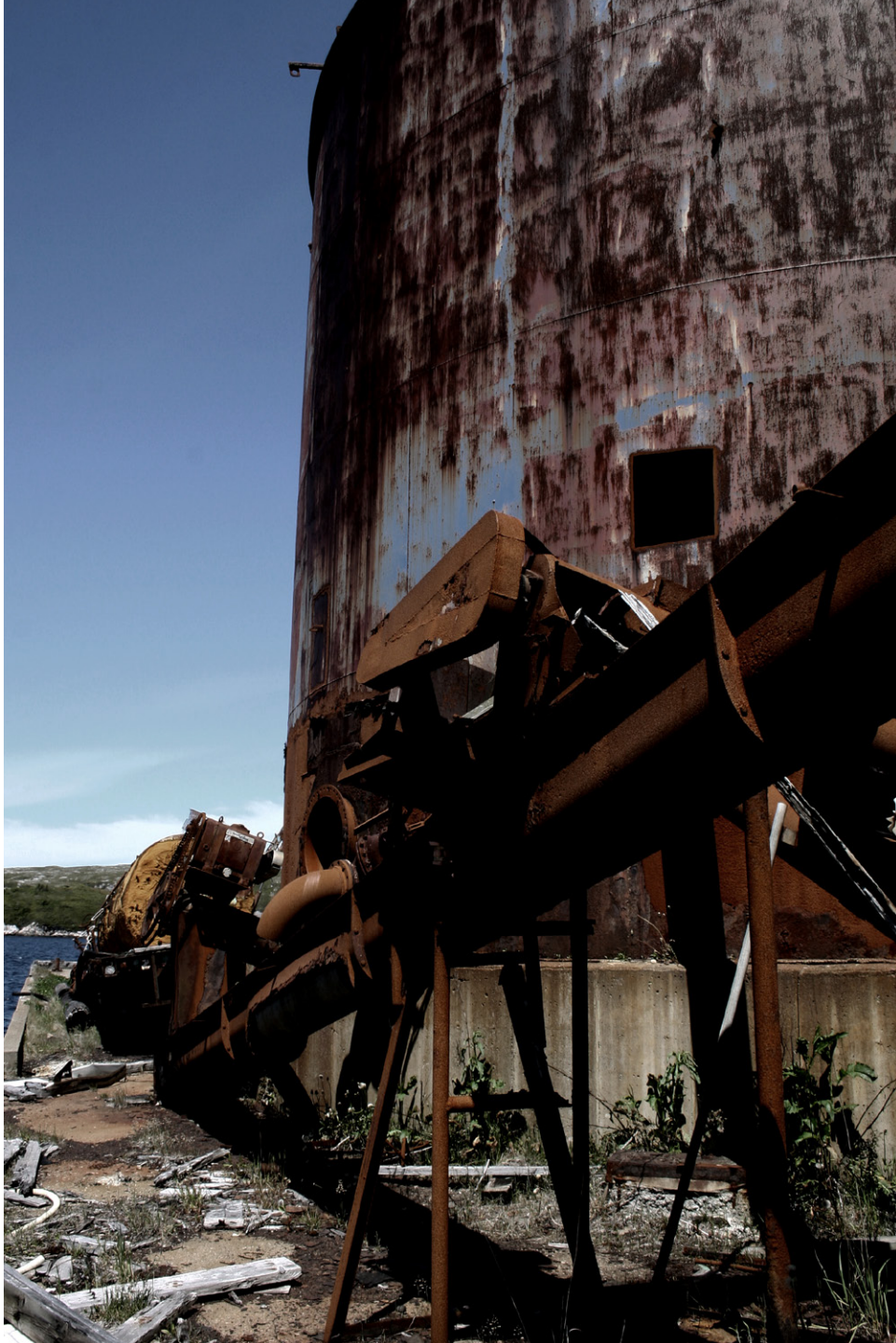
Fig. 1.31 Exterior of storage silos.
