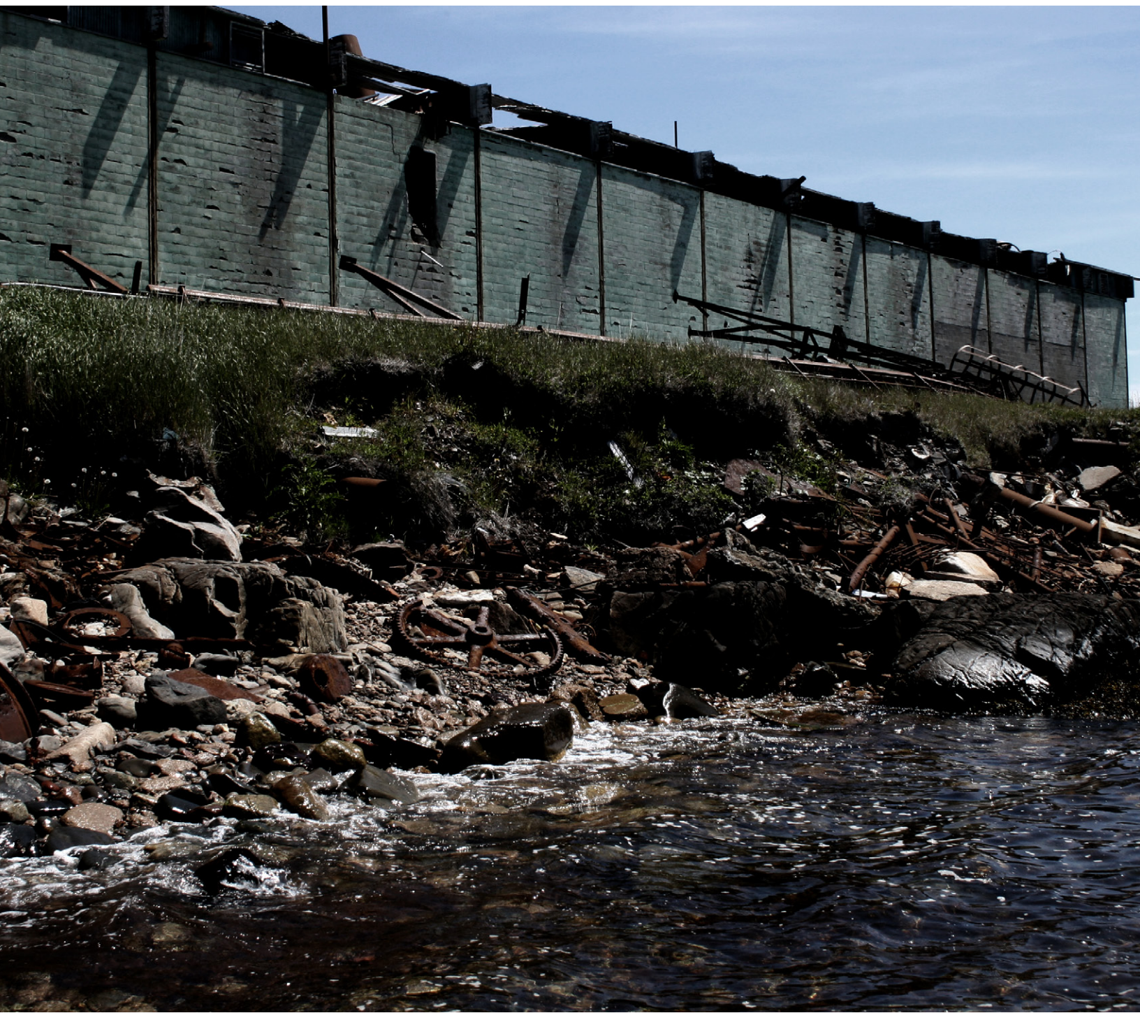
Fig. 1.33 Second plant building.
