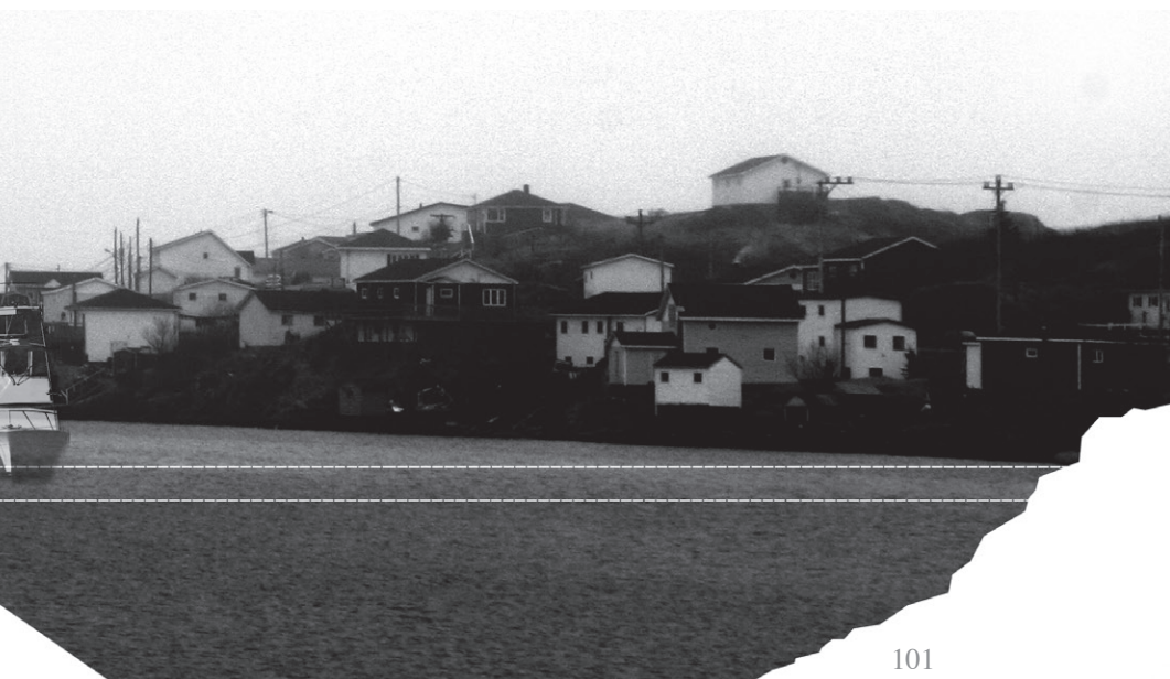
Fig. 2.10 Burgeo Facility Sections : Degrees of interaction with the elements. Ranging from Resist, Converse, Surrender.
