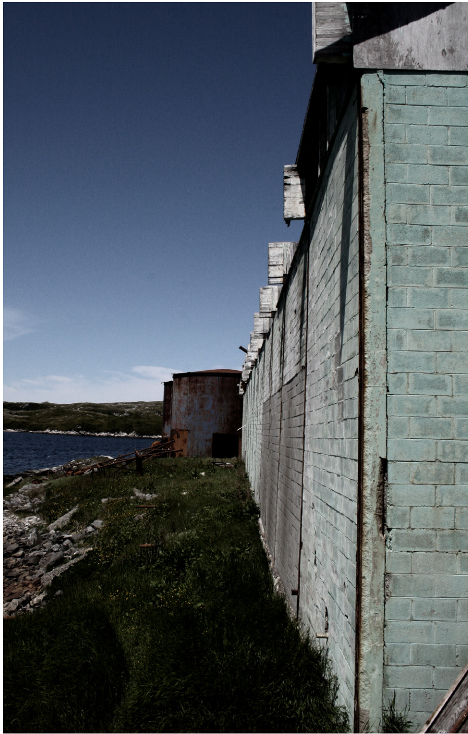
Fig. 1.34 Second building with storage silos in background.
