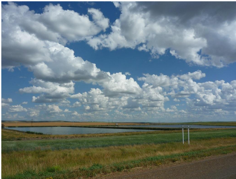
Figure 26 Two cell sewage lagoon in Coronach
