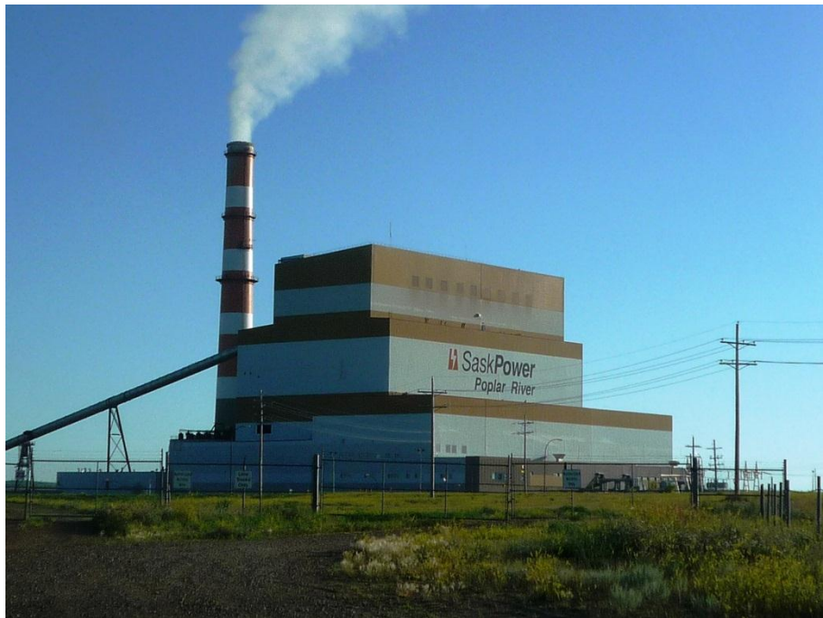
Figure 30 SaskPower Poplar River Power Station
