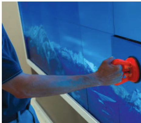
Figure 17 c : Micro Tiles Easy Wall Installation and Services
