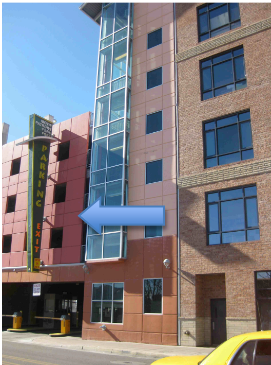
Image 5-4: Parking Structure (Available for private use by residents of the Gold Street Lofts and for public use for a small fee.)
