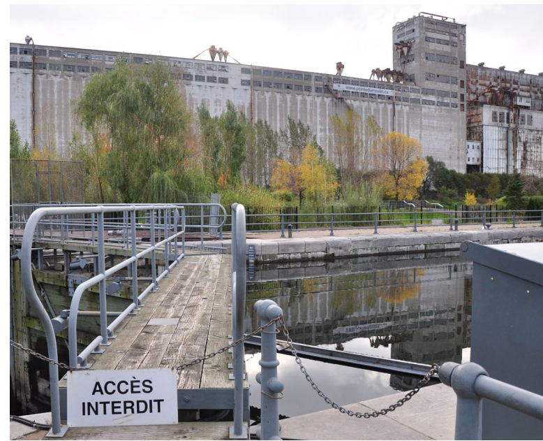
fig.2.3.6 Lock 1 on the Lachine Canal in a semi-closed position limits the water flow through the canal to near stagnant. The locks and canal edges are inaccessible in this basin, though further along the canal moving away from the city centre, Côte St. Paul lock and St. Gabriel lock are traversable.
