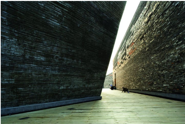
fig.4.1.9 Ningbo History Museum recycled material facade.
