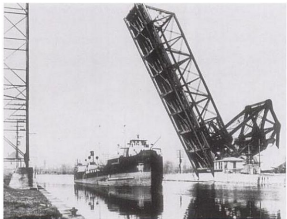
fig.1.1.5 Image of the 'Jackknife' Lift Bridge over the Lachine Canal.
