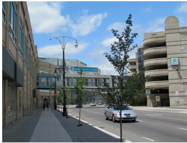
Figure 16: “Plus 15” Overhead route between the former Eaton Centre and Parking Garage, York Blvd
