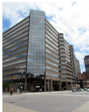
Figure 124: Standard Life Centre, Bay Street North and King Street West
