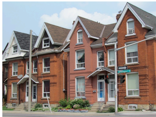
Figure 99: Semi-Detached Homes, Wellington Street North near Wilson Street
