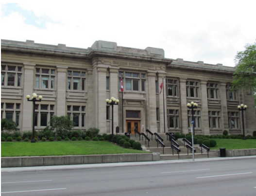
Figure 114: Provincial Court House, Main Street West
