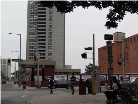
Figure 108: Construction Scaffolding, Main Street East and John Street South
