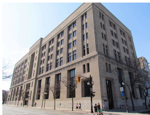
Figure 115: Courthouse, Main Street West and John Street South
