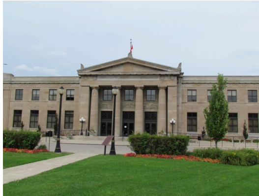
Figure 50: Liuna Station Banquet and Convention Centre, James Street North
