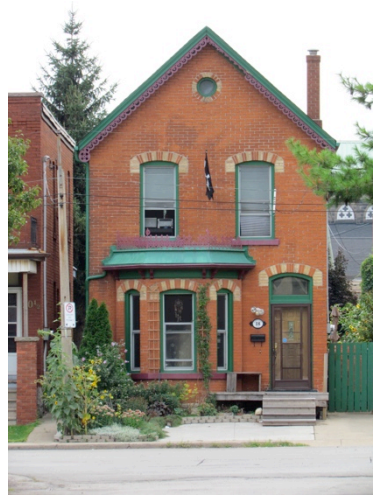
Figure 97: Single Detached House, Murray Street East near Hughson Street North
