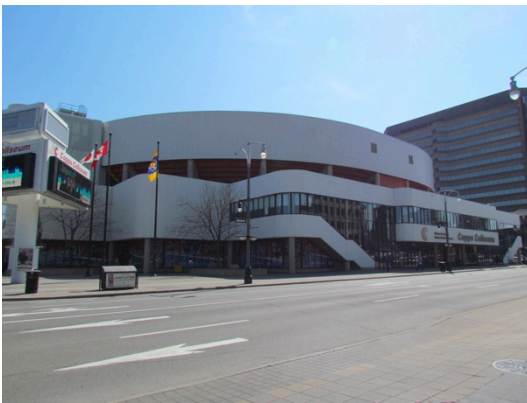
Figure 19: Copps Coliseum, Bay Street North and York Blvd
