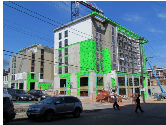
Figure 109: Construction in Progress, George Street and Caroline Street South
