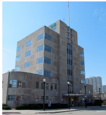
Figure 113: GO Station, Hunter Street East
