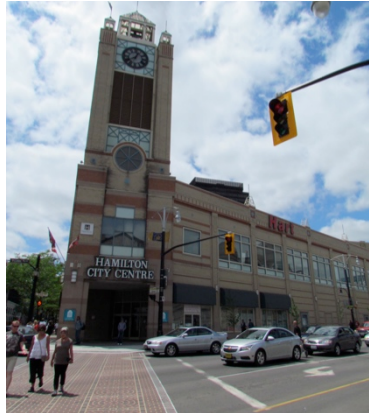
Figure 17: The Former Eaton Centre (now called the Hamilton City Centre), York Blvd
