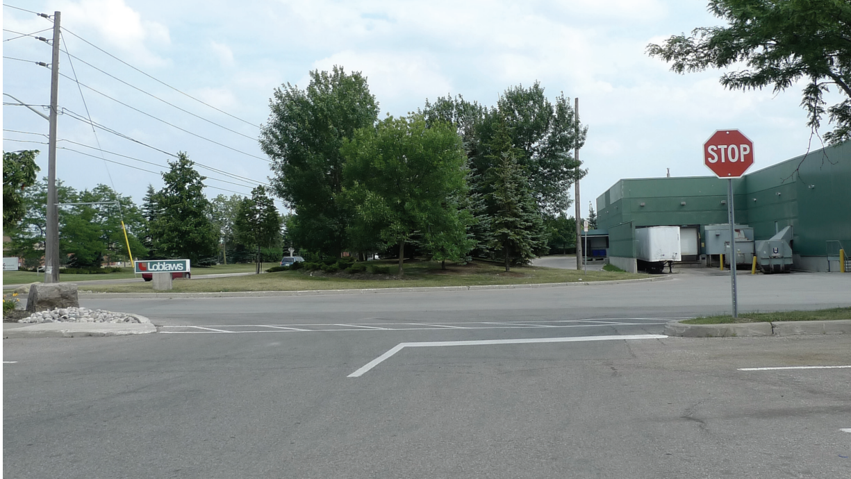
Fig. 36. Loblaws back-of-house and loading area A bland and unwelcoming back-of-house area where trucks load, faces McLaughlin Rd., a major artery into the Loblaws block and the HTC at large.
