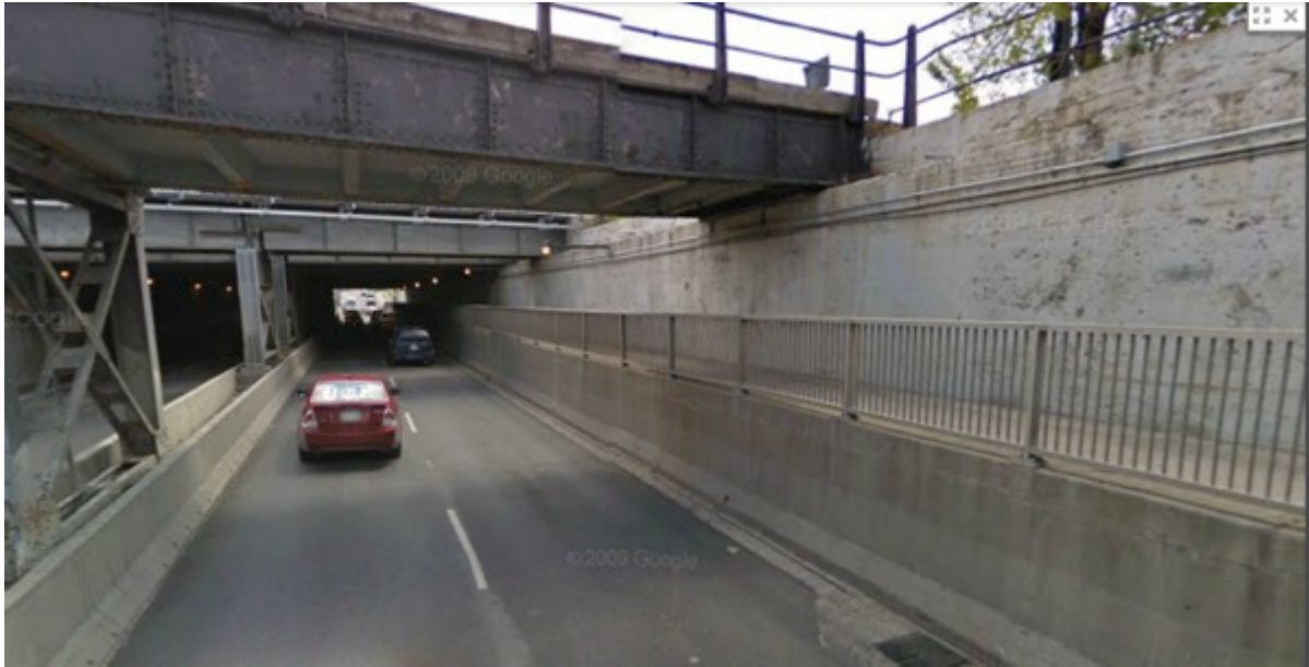
Figure 6-6: Broad Street Underpass (Google Maps, 2012)
