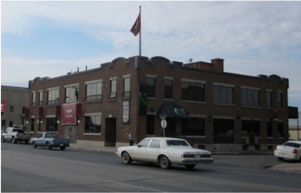
Figure 5-8: Warehouse Partially Converted to Office Use
