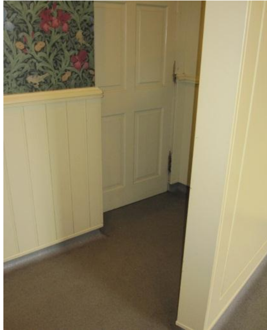
Figure 19. Public washroom entrance from inside.
