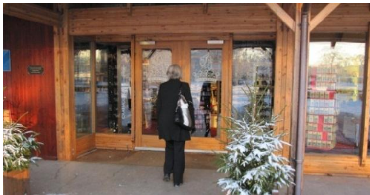
Figure 22. Entrance to gift shop, no automatic door opener (Barlow, 2011).
