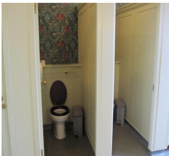
Figure 20. View of stalls inside public washroom (Barlow, 2011).
