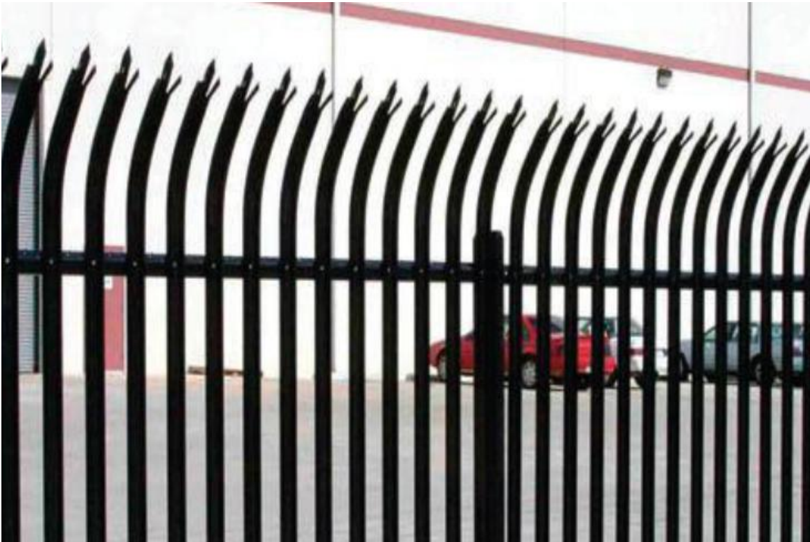
Figure 9: Fences, including this anti-climb example are passive security measures which can make an asset unreachable to foot or vehicle effectively protecting them and forcing attacks to find other way around it including past security points Source: FEMA 430
