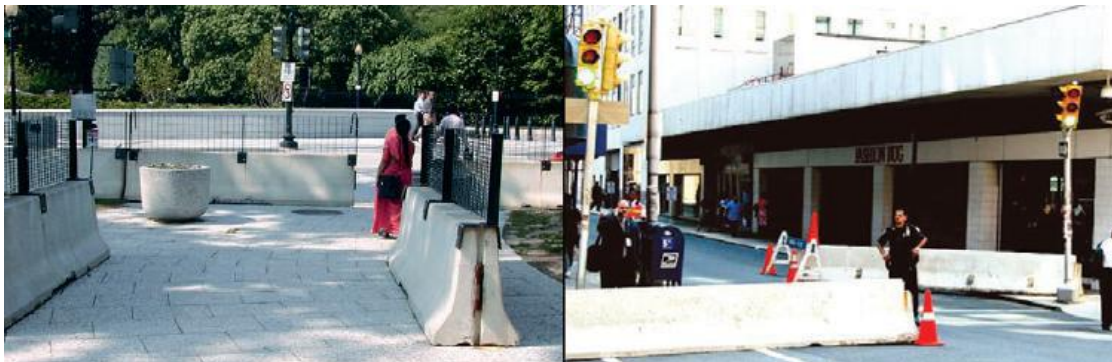
Figure 7: Jersey Barriers are rapidly deployable concrete barriers which can be used to bar traffic and people. They can be bare as seen on the right or with a fence attachment as seen on the left. They can also be used as temporary measures in events which demand it such as a visit from head of state.
