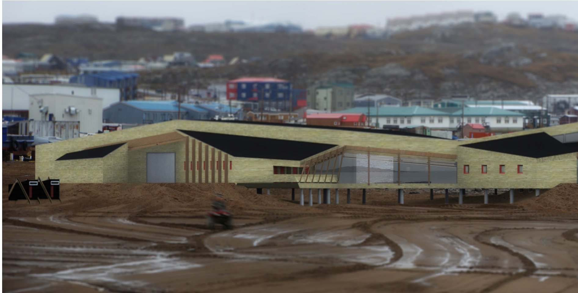
Fig. 4.20 The southern facade of the Nakasuk Facility is clad with large expanses of glazing to capture passive solar heat and to offer uninterrupted views of Koojessee Inlet.
