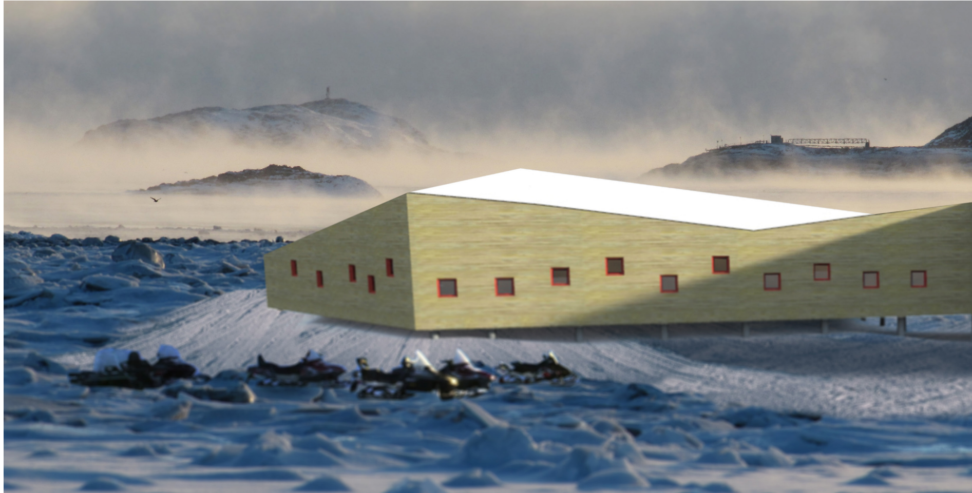
Fig. 4.25 The northern facade of the Nakasuk Facility harmonizes with the surrounding rock formations. Given that prevailing winds batter this facade, minimal glazing is used to help with heat retention. The only exception is a single window in the center which acts as a lens from which to view the natural landscape beyond.
