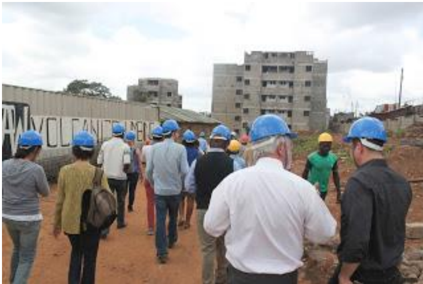
Figure 6.2: Soweto East Redevelopment in Progress (G, 2013)
