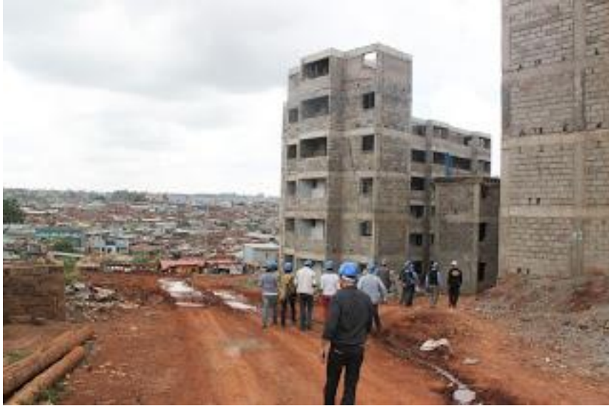
Figure 6.1: Soweto East Redevelopment in Progress (G, 2013)
