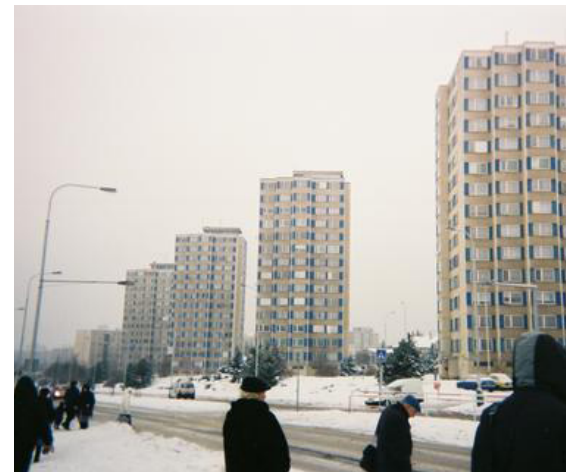
fig. 2.61 | Behind the Iron Curtain: Soviet era Panelák , or 'panel tower houses' in Prague
