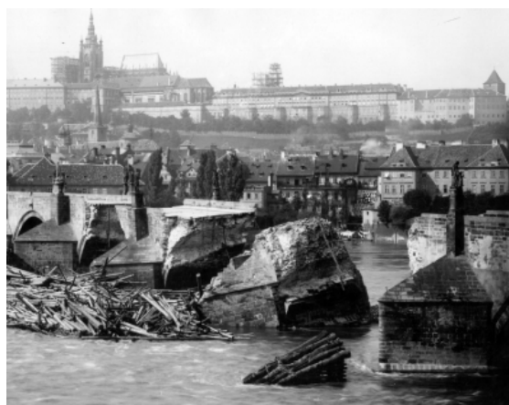
fig. 2.47 | Aftermath of 1890 flood
