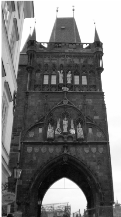
fig. 2.42 | Old Town Bridge Tower
