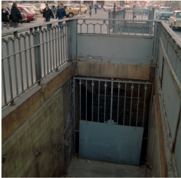
fig. 3.47 | Closed U-Bahn Stadtmitte Station in East Berlin
