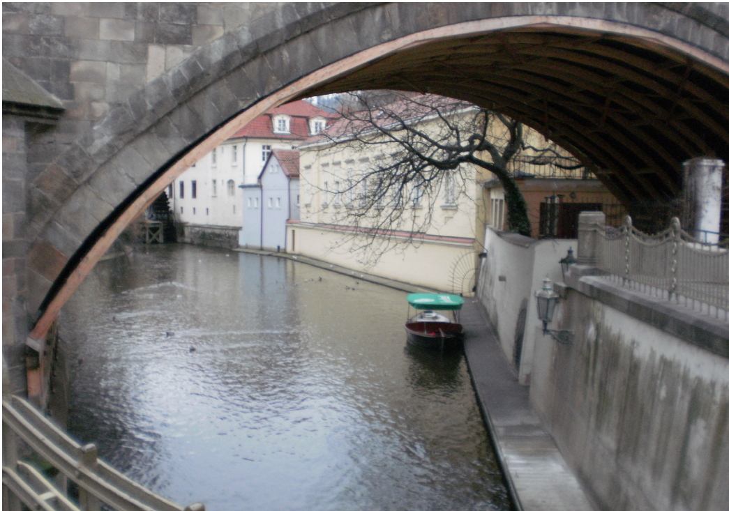
fig. 2.49 | Arch detail at Kampa Island on Lesser Quarter side
