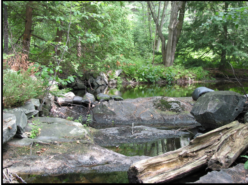
Figure 4.3.4 – Bass Lake Rock Weir
