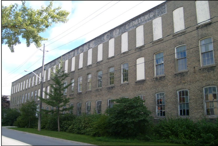
Figure 24: Example of Older Industrial Building with Original Wood Windows
