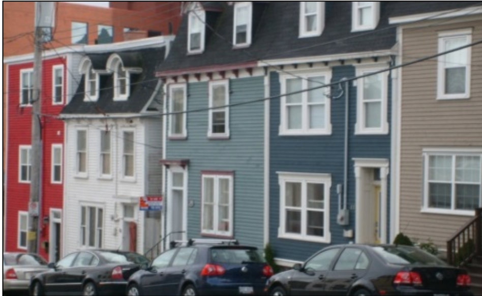
Figure 1: Example of Window Replacement, St. John's, NL
