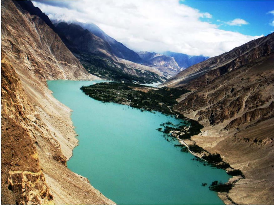
Figure 2.12: Aerial view of 2010 Hunza rockslide-dammed lake in northern Pakistan. At the time of the photograph (May 13, 2010; day 127 of impoundment) lake waters are still rising (pool el. 2,423 m a.s.l.), filling the Hunza Valley. View is upstream. Lake would rise another 12 m before overtopping on May 29, 2010 [Pamir Times photograph].
