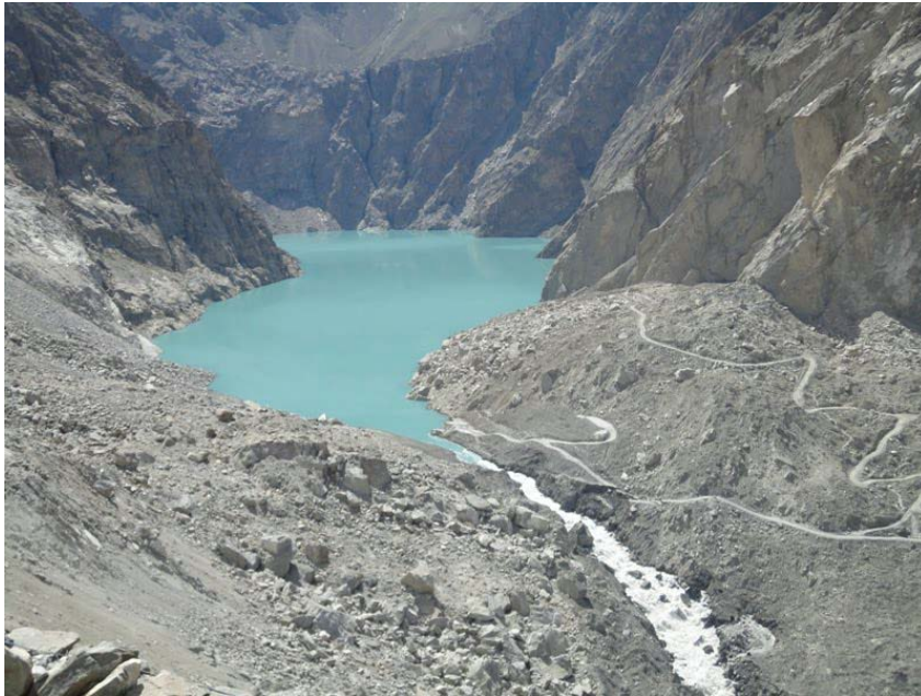
Figure 2.15: View of overflow of 2010 Attabad rockslide dam and the Hunza rockslide-dammed lake in the background. Date of photograph is June 10, 2010 12 days after overtopping on May 29 (143 days after impoundment). Volume of lake is ca. 430 Mm 3 . Note limited erosion of spillway. Photograph by Focus Humanitarian Assistance, Pakistan.
