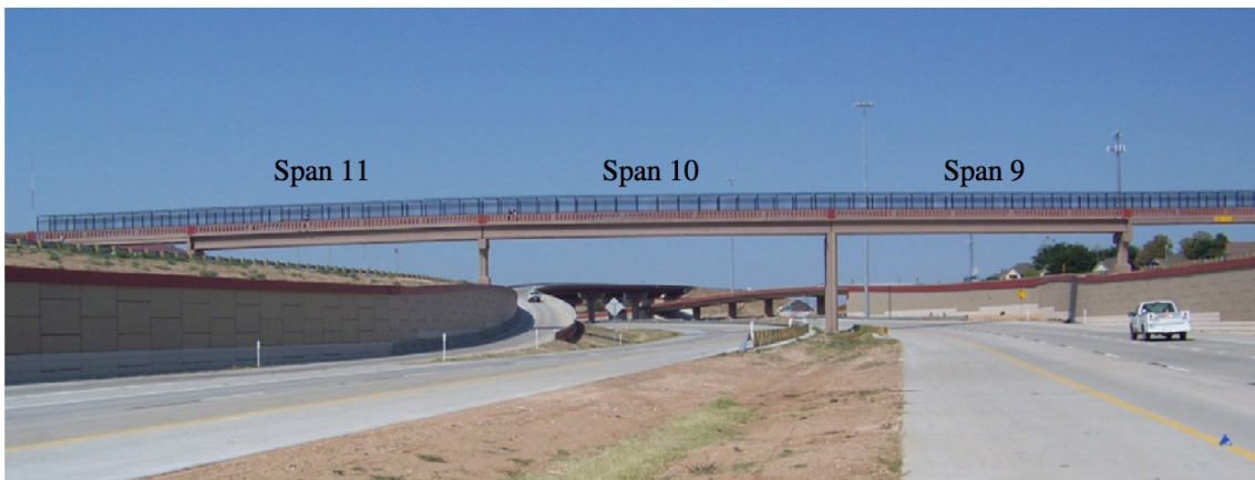
Figure 2.4: Pedestrian bridge at Texas Tech University, USA (106)
