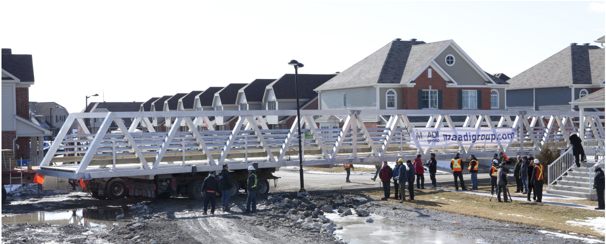
Figure 1.1: Installation of light-weight aluminium bridge (86)
