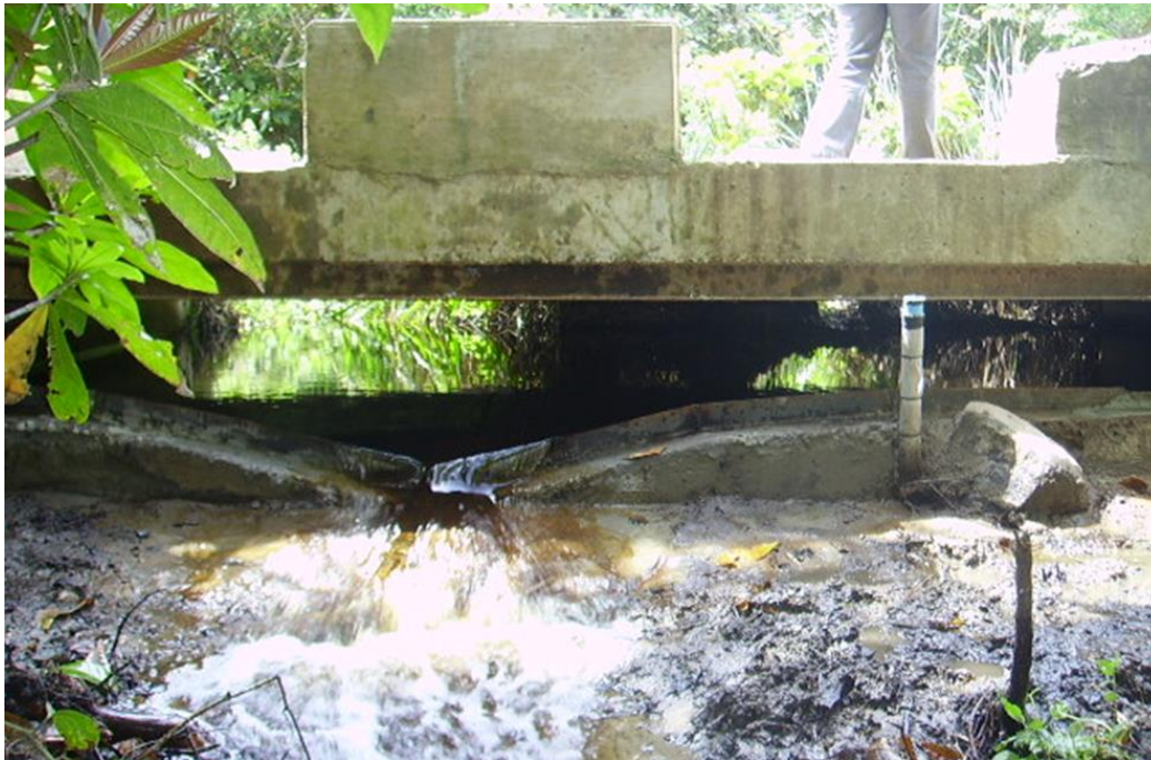
Figure A2: The Nkazana stream measuring weir – a compound weir. Note the wide angle of the V-notch.
