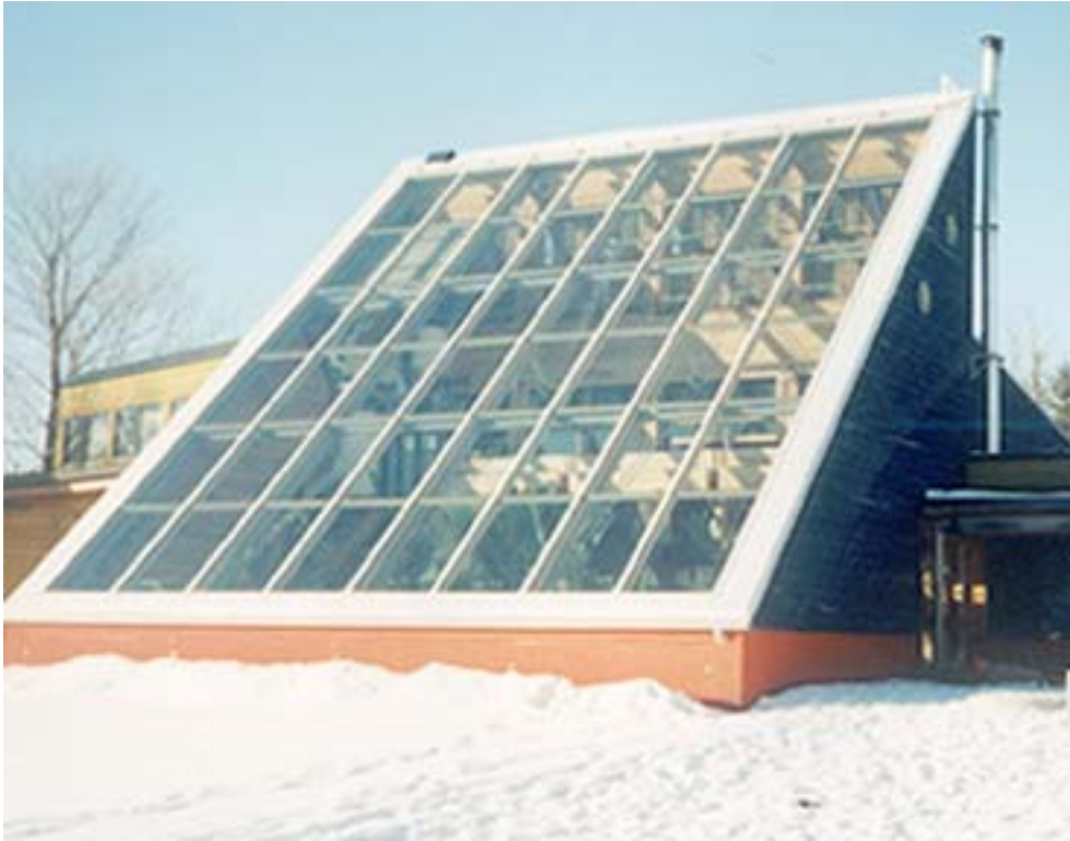
Figure 5-2. YMCA Greenhouse enclosure.
