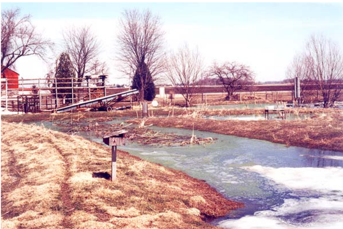
Figure 4-4. Constructed treatment wetland during (spring melt 2001).
