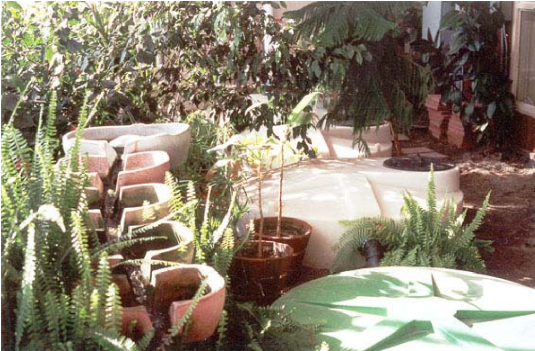
Figure 5-8. Greenhouse-based treatment technology: Flowform and closed aerobic reactors.
