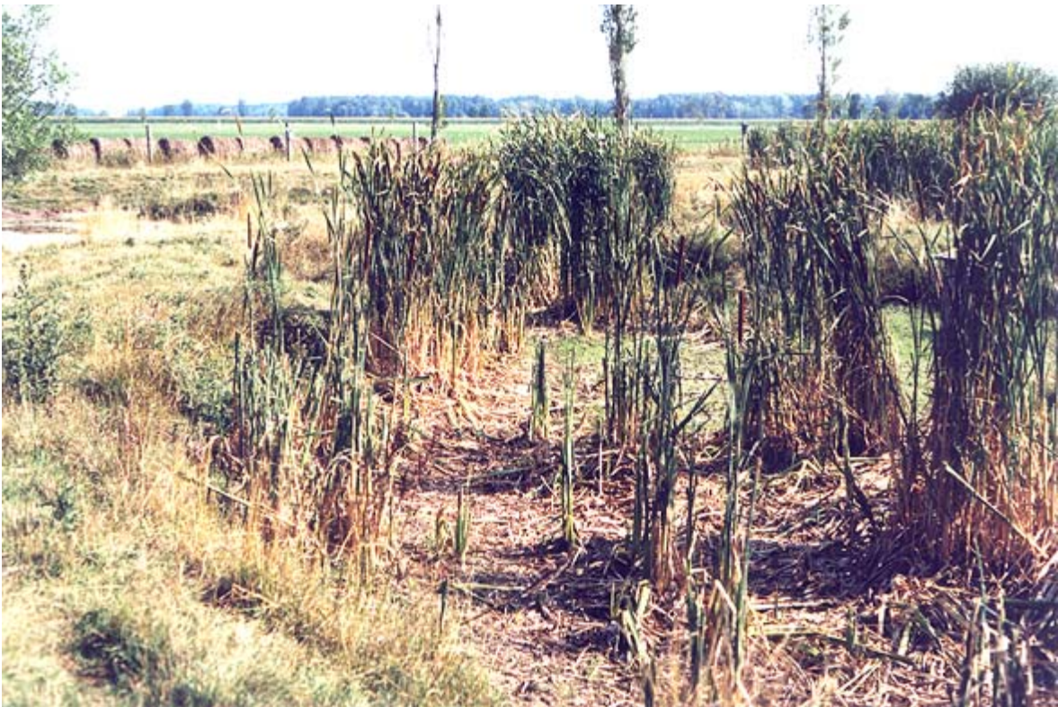
Figure 4-6. Constructed treatment wetland (drought of 2000).
