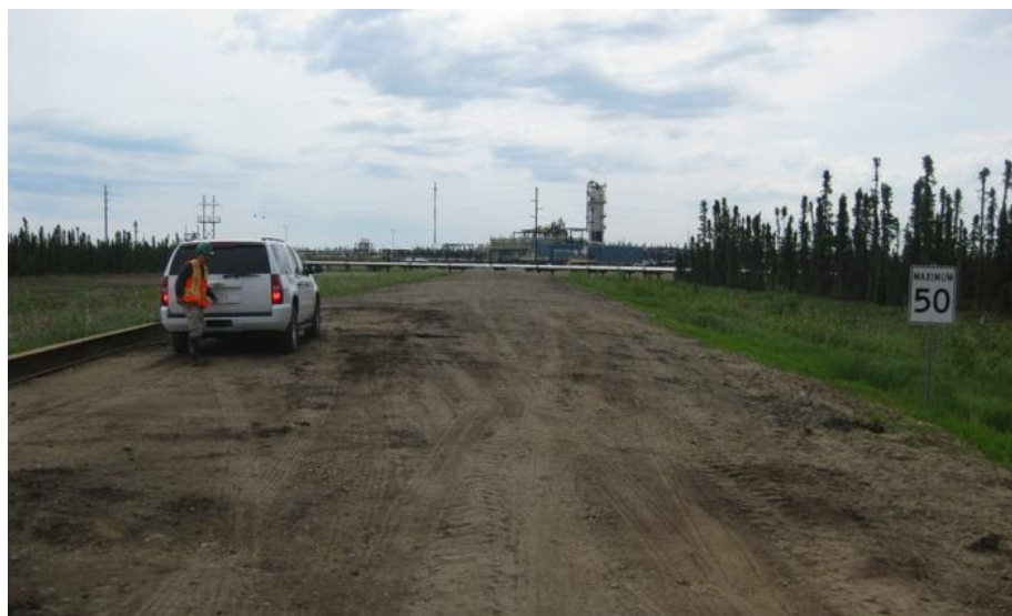
Figure 2-2. Suncor Firebag Site Aerial photograph 2013 with Pad 106 Access Road circled in yellow and photograph taken from the access road. Pad 106 Access Road was a small road that was cut off from Pad 106 by an above-ground pipeline. (Source: Suncor, Corey Vogel, 2013)
